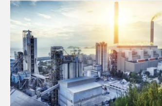
Factories need H24 electricity supply
